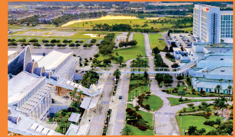
HILTON PEDESTRIAN BRIDGE
